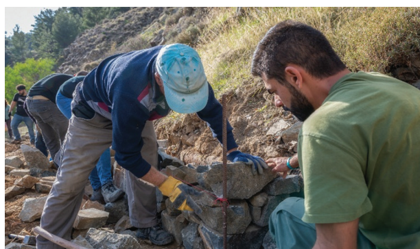
Construction of drystone walls
