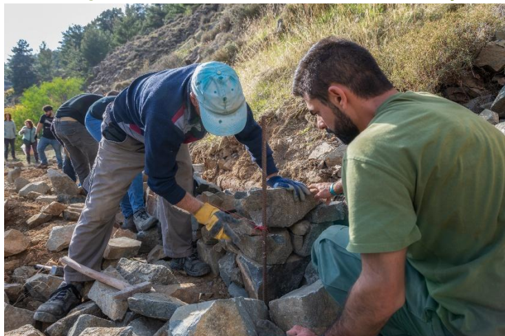
Figure 12: Construction of drystone walls
