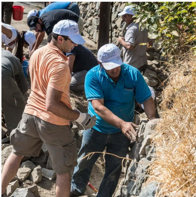
Stakeholders restore collapsed dry-stone terrace walls following instructions given by experts. (Christos Zoumides)
