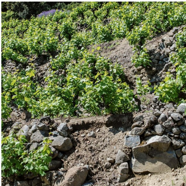
Collapsing dry-stone walls (Christos Zoumides)
